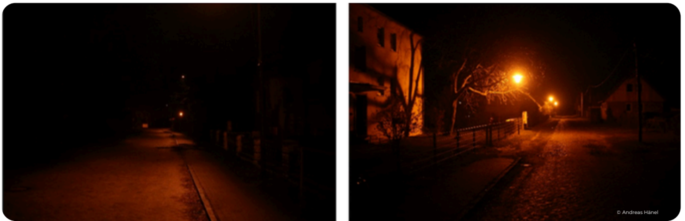
Figure 17: The effect of specially tailored luminaires, that direct light only to the area to be illuminated compared to the old installation (right) in the same street (AUBE project in Nature Park Westhavelland, source: A. Haenel).
