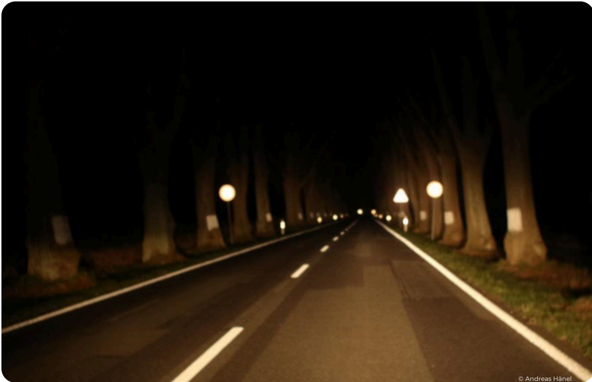
Figure 11: Good reflective markings allow to recognize the course of a street very well without additional installed artificial light (Source: A. Haenel).
